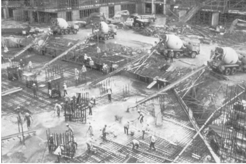
FIGURE 42.3 Concrete placing at Raffles City, Singapore.
